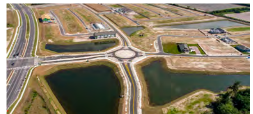
▲ Waterset Phase 4, Hillsborough County
