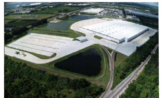
▲ Home Depot Distribution Center, Hillsborough County, FL
